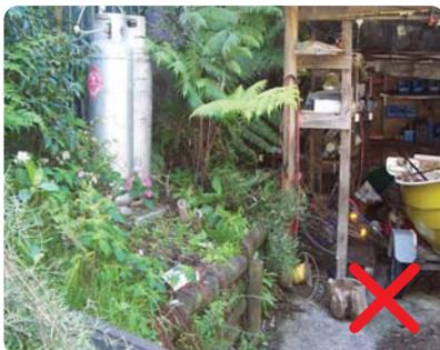
Cylinder installations should be in an accessible location where the delivery of gas can be made safely by one person.
