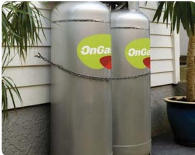
The access route should be clear of obstacles and not be over delicate or decorative surfaces such as terracotta due to the weight of the cylinders.
